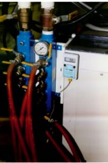
This E-Z Probe® is mounted using the magnetic backing.
