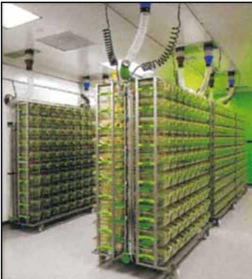
IVC rack integration into HVAC System
